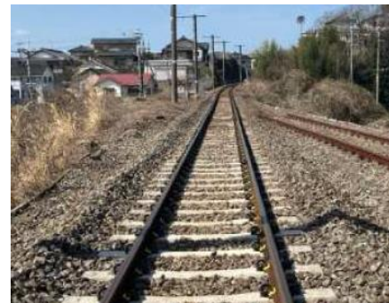
Promoting the use of TCP sleepers
