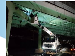
Comprehensive maintenance of overpass bridges
