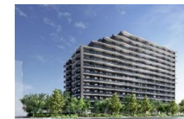
RJR Precia Higashi Jujo Garden (Completed in February 2025)
