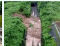
Collapse of cut slopes
