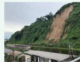
Collapse of cut slopes
