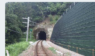
Retaining wall using the “geo rock wall construction method”
