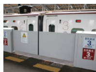
Platform screen doors on Shinkansen platform
