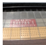
Tactile pavement tiles with a line to indicate the safe side of platform
