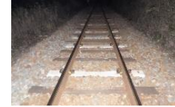
Transitioning to TPC railroad ties
