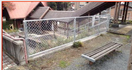
Installation of fence to prevent falls
