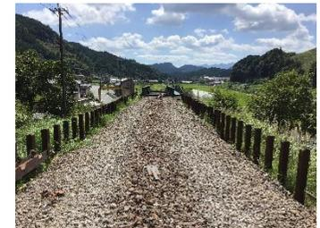
Rails from the track were cut and driven into the ground as earth retaining piles for the dedicated road, and the ballast was mixed with gravel and reused as a base for the pavement.
