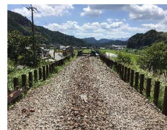
Rails from the track were cut and driven into the ground as earth retaining piles for the dedicated road, and the ballast was mixed with gravel and reused as a base for the pavement.
