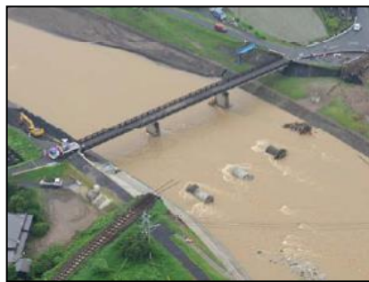
■ Washed away Kagetsugawa Bridge between Teruoka Station and Hita Station, Kyudai Line (left) and reconstructed site in April 2018 (right)
