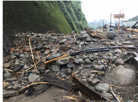
■ Sediment runoff on the premises of Chikuzen-Iwaya Station, Hitahikosan Line
