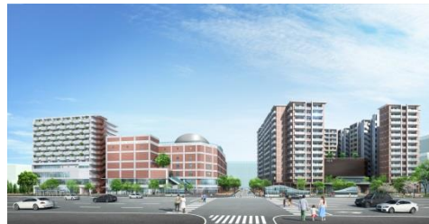
■ Ropponmatsu development project
