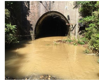
■ Sediment runoff on the Nippo Main Line between Tsukumi Station and Hishiro Station
