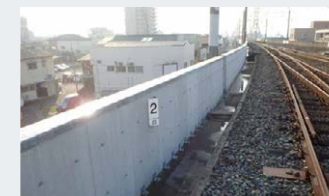
Elevated bridge using the “smooth board construction method”
