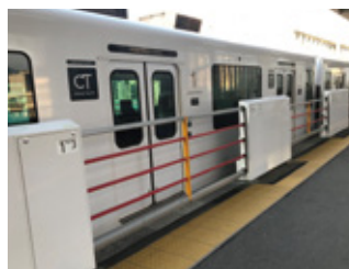
Platform screen doors (Chikuhi Line)
