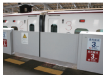
Platform screen doors on Shinkansen platforms
