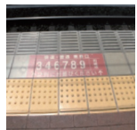
Tactile pavings with a line to indicate the safe side of platform
