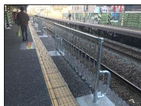
[ホーム固定柵(笹原駅)]
